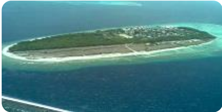
Dharavandhoo Airport, Baa Atoll
